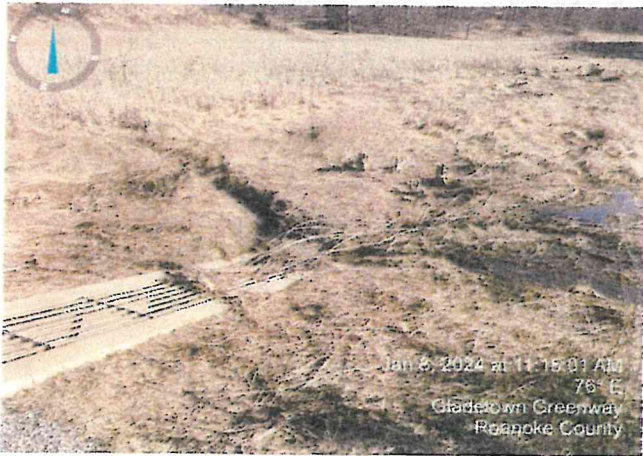
Remove woody debris and trash from the low flow grate.
