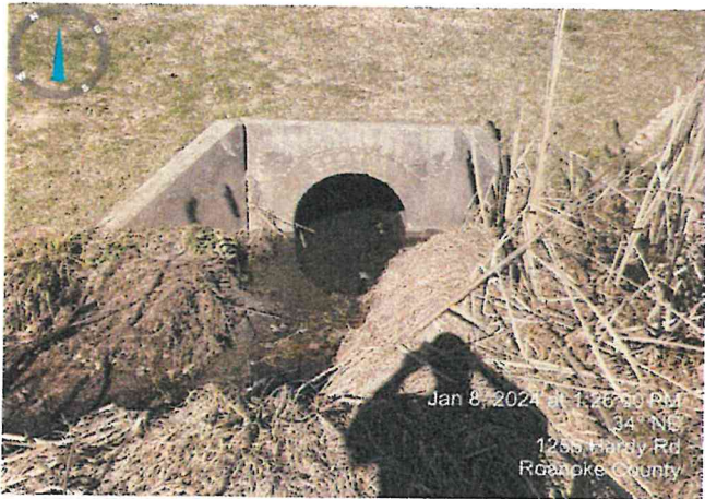
Remove accumulated sediment and debris from within and below the inflow pipe. Install outlet protection once the accumulated sediment has been removed.
