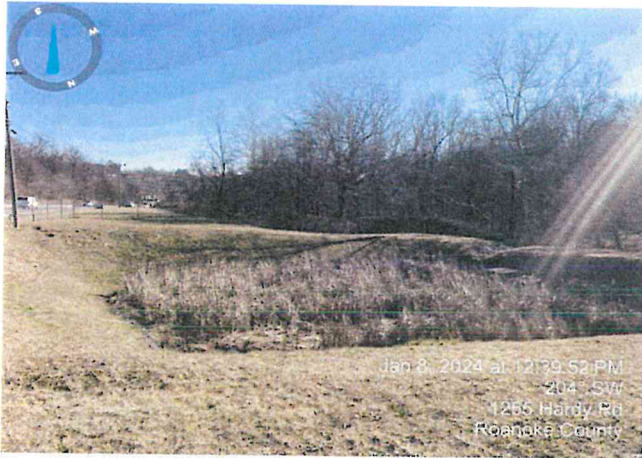
Remove accumulated sediment and grade to ensure positive drainage from the inflow to the outlets.
