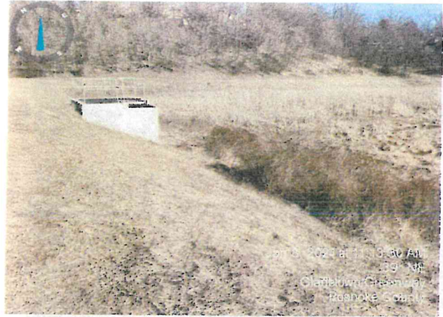
Remove woody growth from the embankment.
