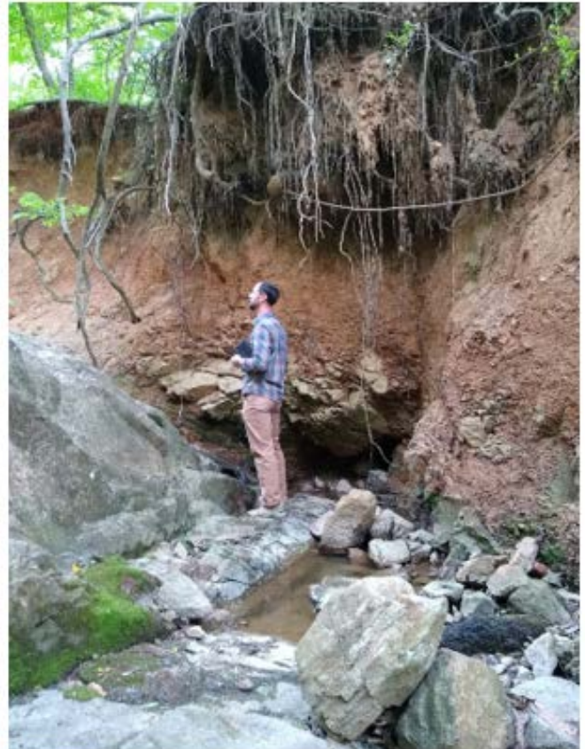
Existing eroding vertical banks along the drainage area at Woodland Place will be restored using the DEQ SLAF and Town's funds.
