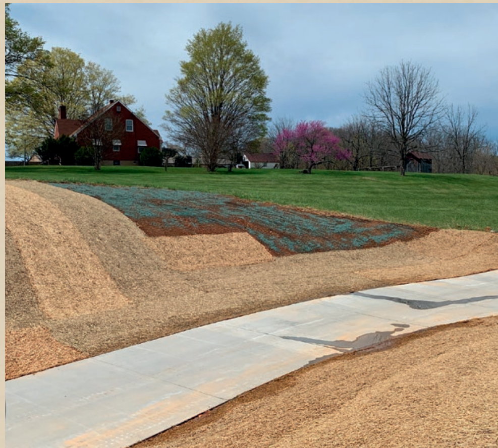
To avoid erosion, cover bare soils with straw mulch, soil retention fabric, sod, hydroseed, stone, or even a plastic tarp. This will protect the soil against highly-erosive wind and raindrop erosion and help to keep the dirt on your project.
