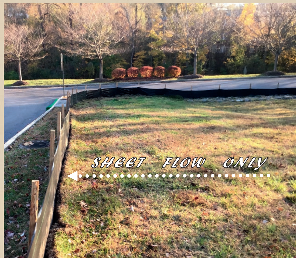
Properly install silt fence by entrenching the bottom of the fabric into the soil. Make sure that the stakes are on the opposite side of the flow (sheet flow only) that is directed to the silt fence. Ensure to remove accumulated sediment when it reaches 1/2 the height of the fabric to avoid over-topping.
