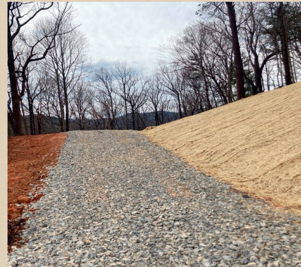
Use VDOT #1 stone, 6" deep, over geotextile fabric for construction entrances. The heavy, angular stone helps knock dirt off of construction vehicle tires, which minimizes sediment tracking onto the road, and the fabric underlayment keeps the stone from getting mired down into the soil.
