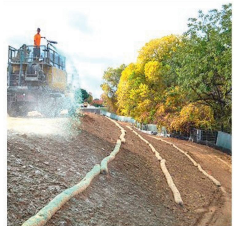
Sediment retention rolls, often called filter socks, are quite effective at slowing the flow of stormwater runoff, which helps to minimize erosion. Once sediment rolls are in place and properly secured, soil protection measures such as straw mulch or blanket/matting are needed to further protect the bare dirt from erosion.
