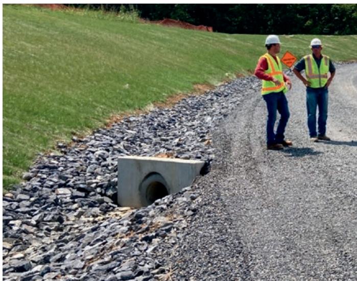
A stable, rip-rap channel will provide excellent erosion control in channels with higher flows.
