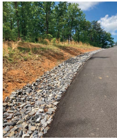
A well-graded rip-rap channel properly keyed in to existing grade.
